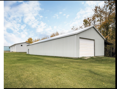
36X80 COLD STORAGE SHED
